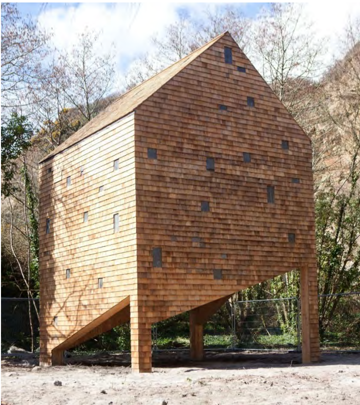
Figure 5-3: Example of a Bat Roost Building: Bat House at Carlyon Bay
